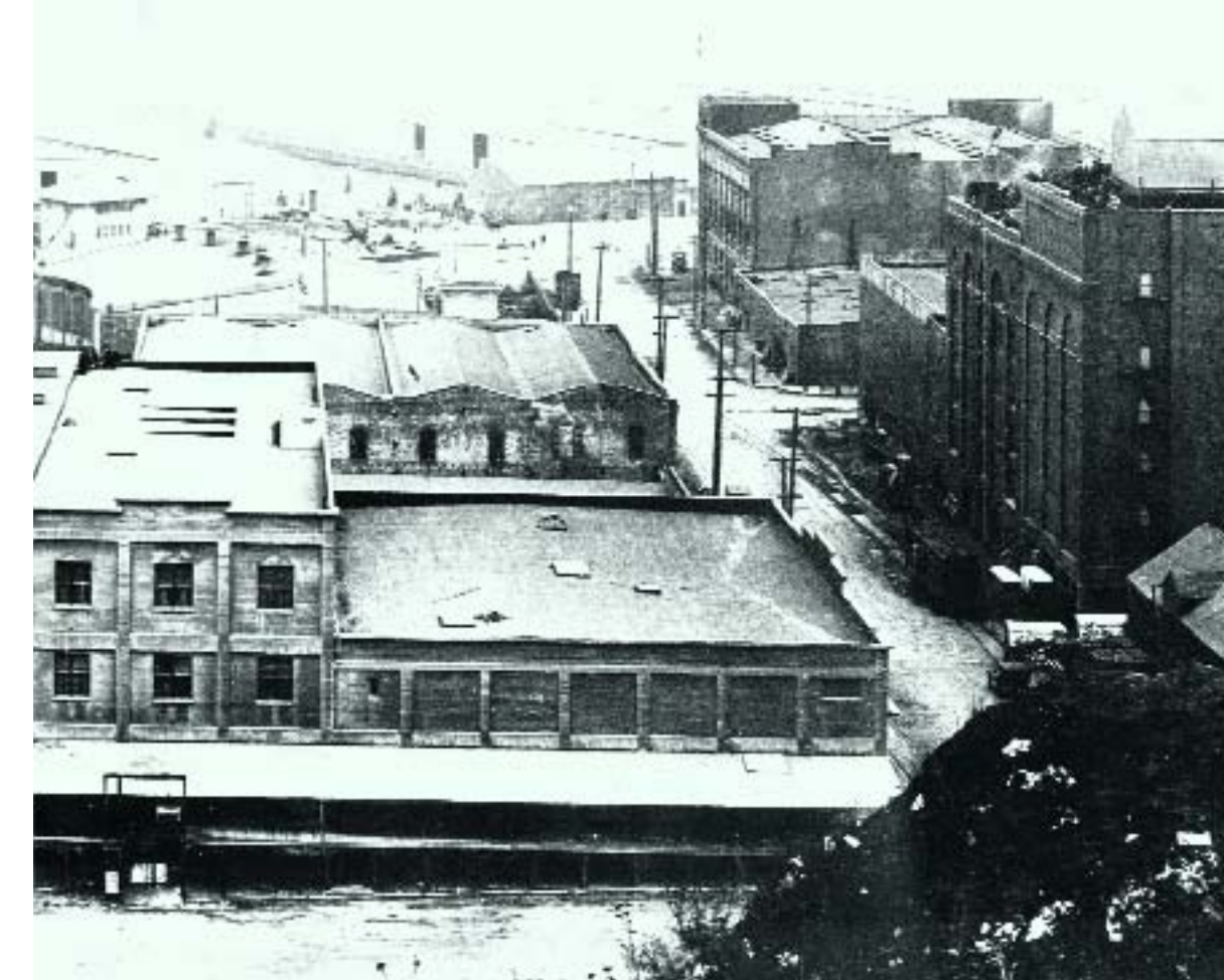
(37) In this shot taken in 1920, we are looking east on Lombard Street and can view part of its intersection with Sansome. One Lombard is in the rear, and a bit of the older Merchants' Ice and Cold Storage buildings are in the right foreground, on this side of Sansome. The left and center of the photograph shows us the old Seawall warehouse building, with the ancient original structure in the background. In the foreground is 1620 Montgomery, the former Del Monte Milling building. The Seawall warehouse was one of the oldest existing warehouses in San Francisco until its demolition in the 1970s.
