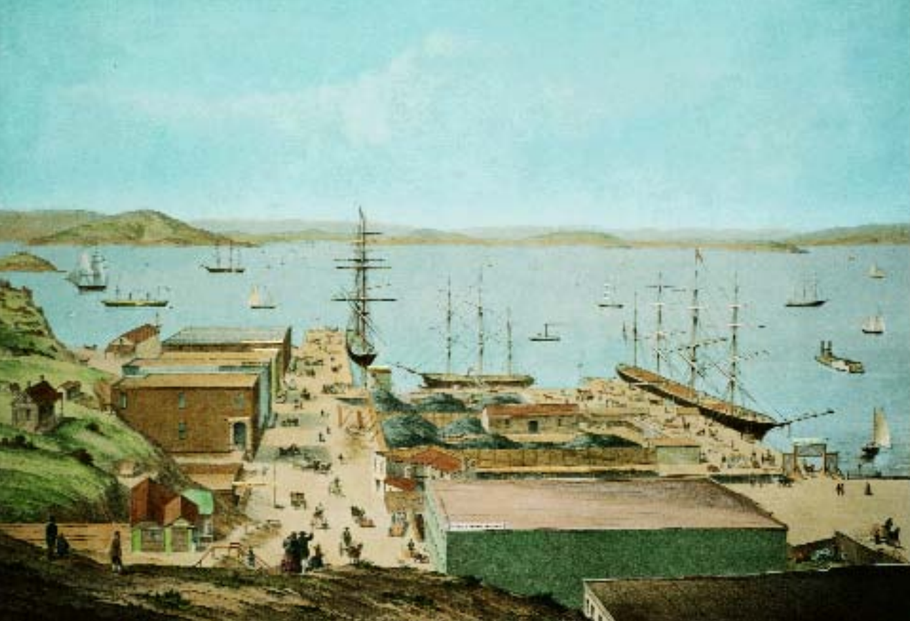
(35) This illustration shows a part of the Old North Waterfront, just a few years into the Gold Rush. Flint's warehouse is in the lower right foreground, near where the Italian Swiss Colony warehouse would later stand. Landfill would eventually expand the shoreline just beyond Flint's, and here the Greenwich Dock warehouse would be built, replaced in 1895 by the One Lombard building.
